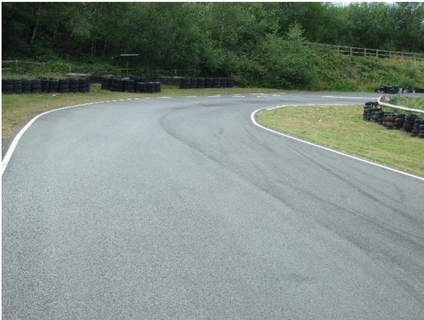
Through Top Pit Bend
